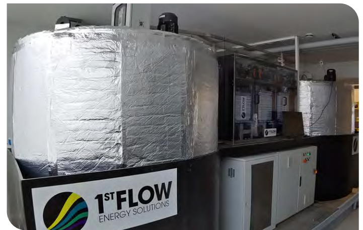
Vanadium redox-flow battery with insulation. (KIT/Felix Schofer)
